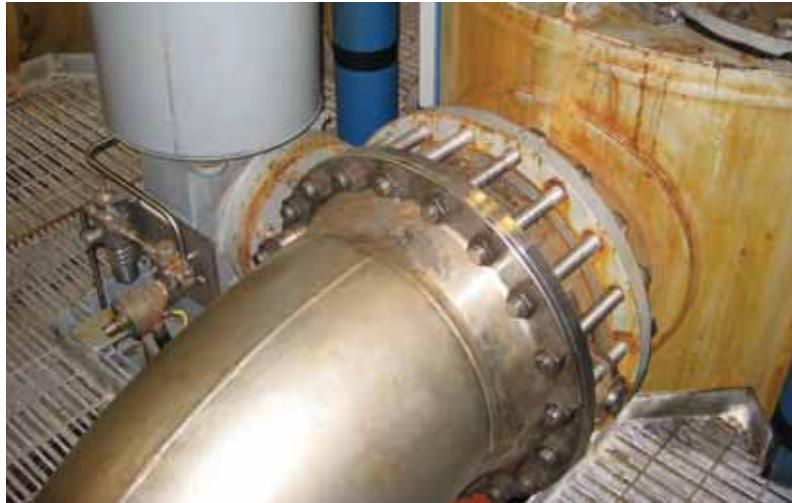
Figure 6.22: Saltwater is one of the most corrosive environments for stainless steel. The main risk is crevice corrosion, and if this is to be avoided, 'super alloys' are required. This cooling water system from an oil rig in the Danish part of the North Sea is made of 4547 (254 SMO). Photo: © Maersk Oil.
