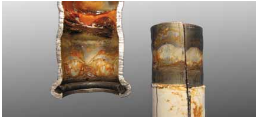
Figure 6.21: Crevice corrosion in press fitting (left) and tubes (right) of 4404 as a result of bacterial growth in tap water installation. The corrosion arose in water with a temperature of 45-50°C with less than 100 ppm of chloride, and it should be noted that the corrosion (the light grey areas on the right) has commenced in the narrowest places where the sleeve has been clamped around the tube.
