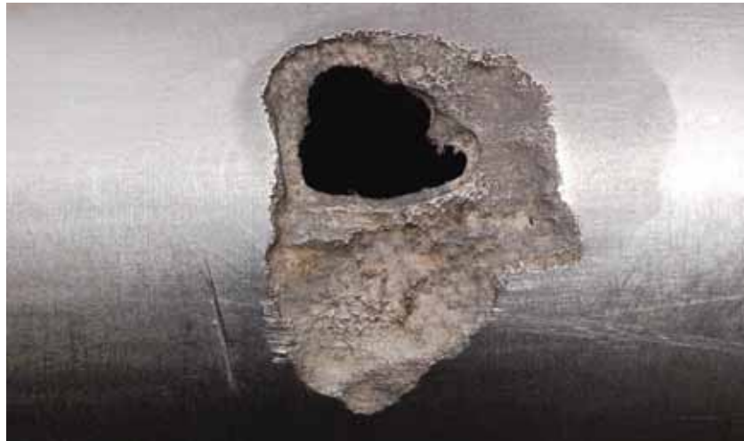
Figure 6.7: Severe penetration in a buried stainless steel pipe (4404) as a result of short distance to a buried, live cable. This has pushed the steel from its ideal passive condition to 'transpassive', and corrosion commences. Note the lack of small corrosion pits.
