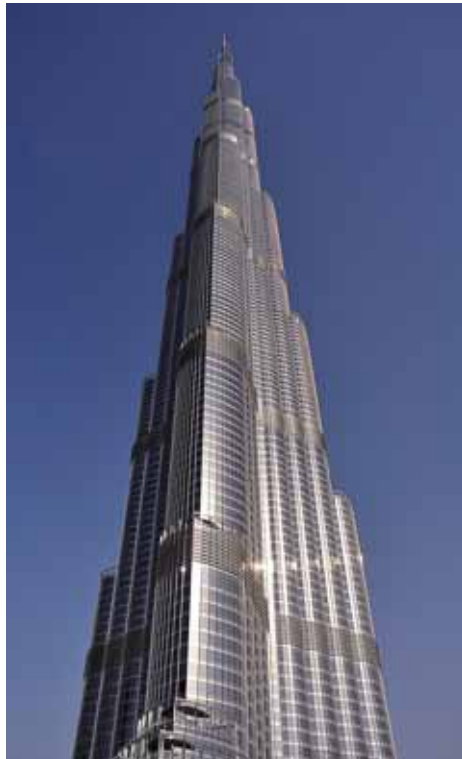
Figure 0.3: With its 828 metres distributed over 162 storeys, Burj Khalifa, located in Dubai, is the world's tallest building and one of its most impressive constructions. Due to the risk of sea salt, large sections of the building are made of type 4404, acid-resistant stainless steel.
