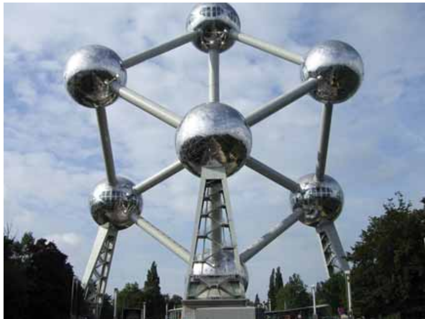
Figure 0.1: Atomium is a Brussels landmark which displays the iron atom's cubic, space-centred structure (BCC). The sculpture is 105 metres high and was originally made in aluminium for the 1958 World Expo. In 2005 the coating was changed to acid-resistant 4404 (1.2 mm plates) supplied by Aperam. Photo: Thomas Pauly, Euro-Inox [11].
